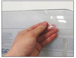
**1.** Peel plastic 4"back on bottom of windshield. Remove completely after windshield is fully installed.
